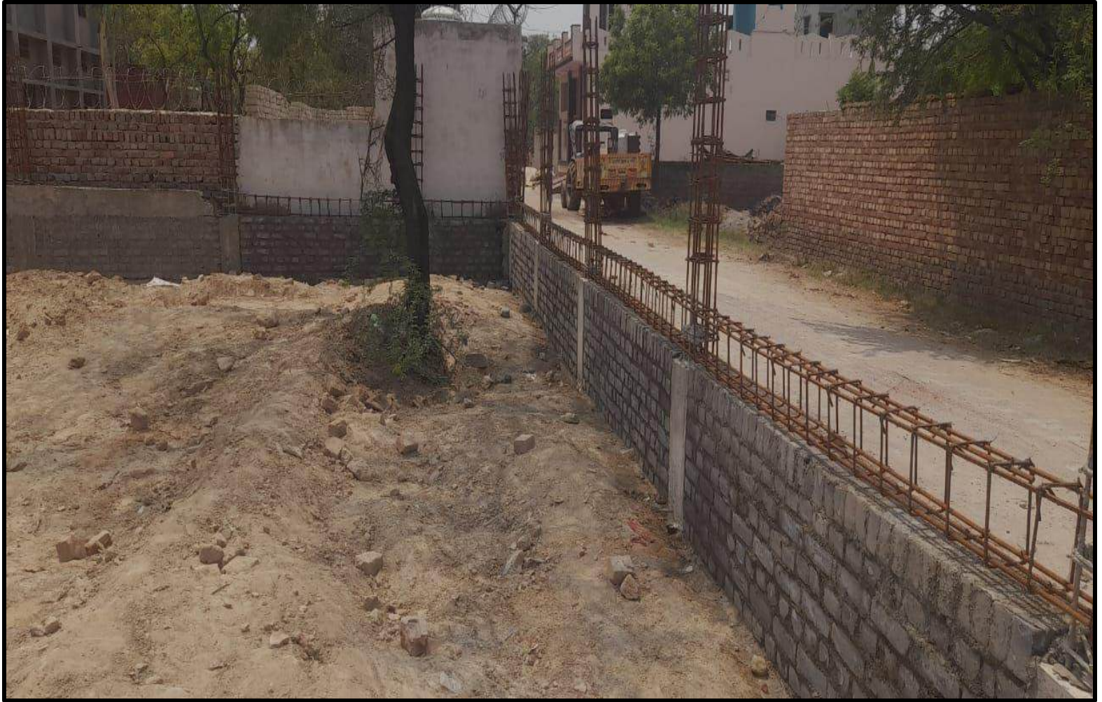
College Boundary Wall Under Construction
