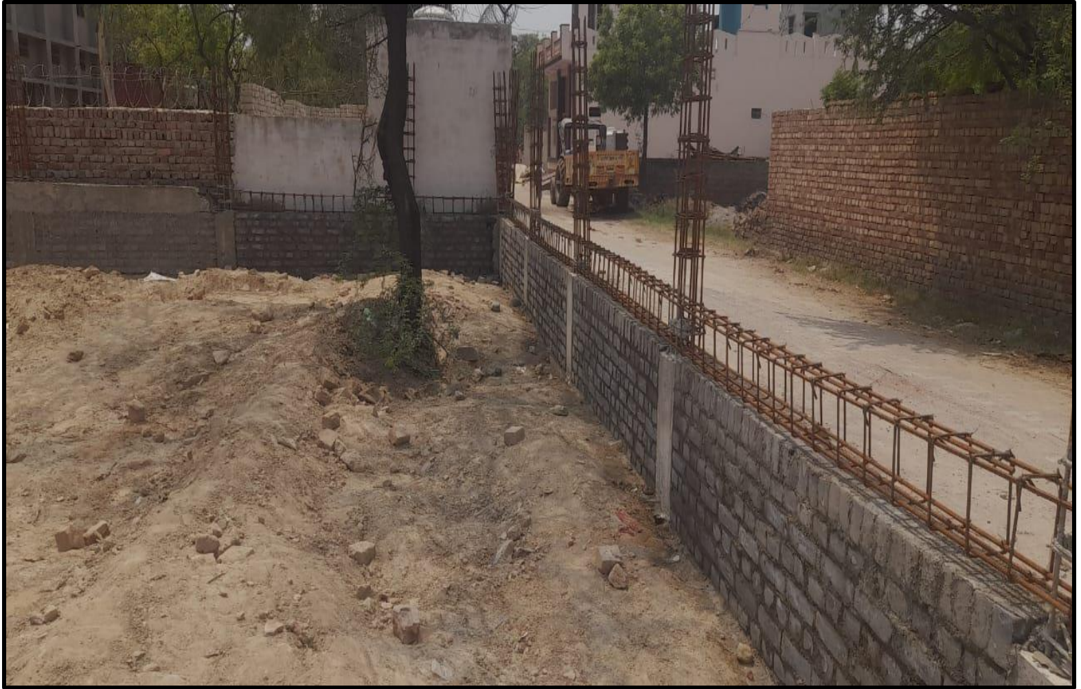
College Boundary Wall Under Construction
